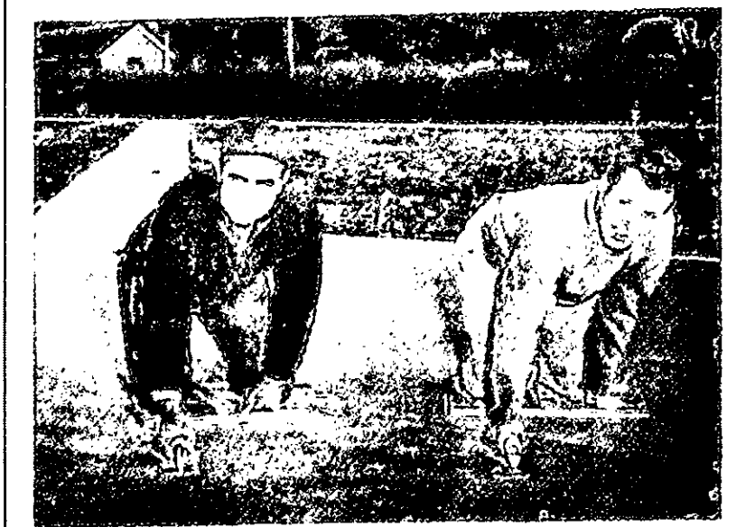
Jaycees Milton Green and Bill Winn (L. to R.) apply their trowels to the last of approximately thirty-nine yards of concrete that the Centerville Jaycees have poured and finished in the past few weeks.
